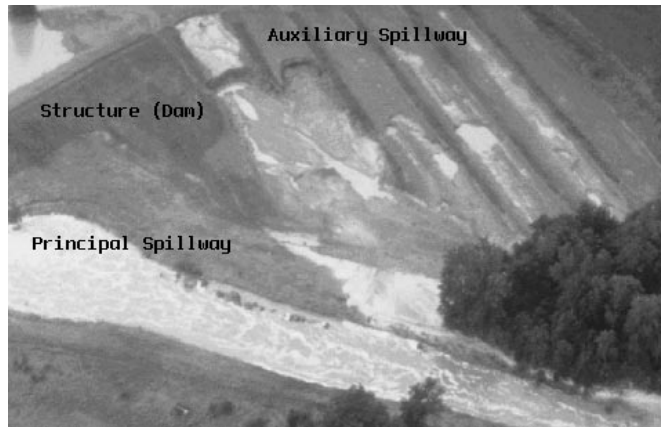
Figure 4: Spillway erosion.
