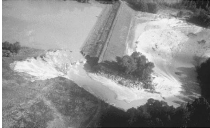
Figure 6: Spillway breach.
